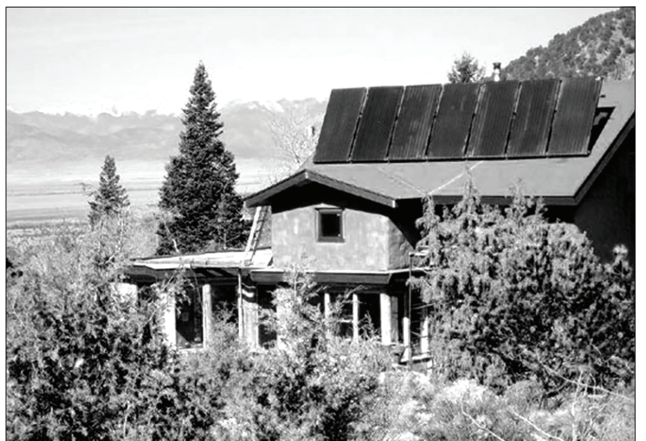
Hybrid passive solar direct-gain home with interior thermal mass walls of rammed earth. Solar thermal panels supply warm water under radiant adobe floor all day for night use. Design/build by Paul Shippee.
