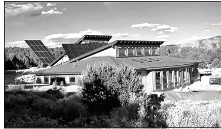
Passive solar Sunspace and clerestory, in Salida, with solar thermal collectors for radiant floor charging and heat distribution. Large, attractive adobe wall between Sunspace and house interiors distributes low temperature daily solar gains at night via large radiant wall areas. This results in hi-performance solar heating approaching 100%. Passive solar design & radiant floor installation by Paul Shippee.
