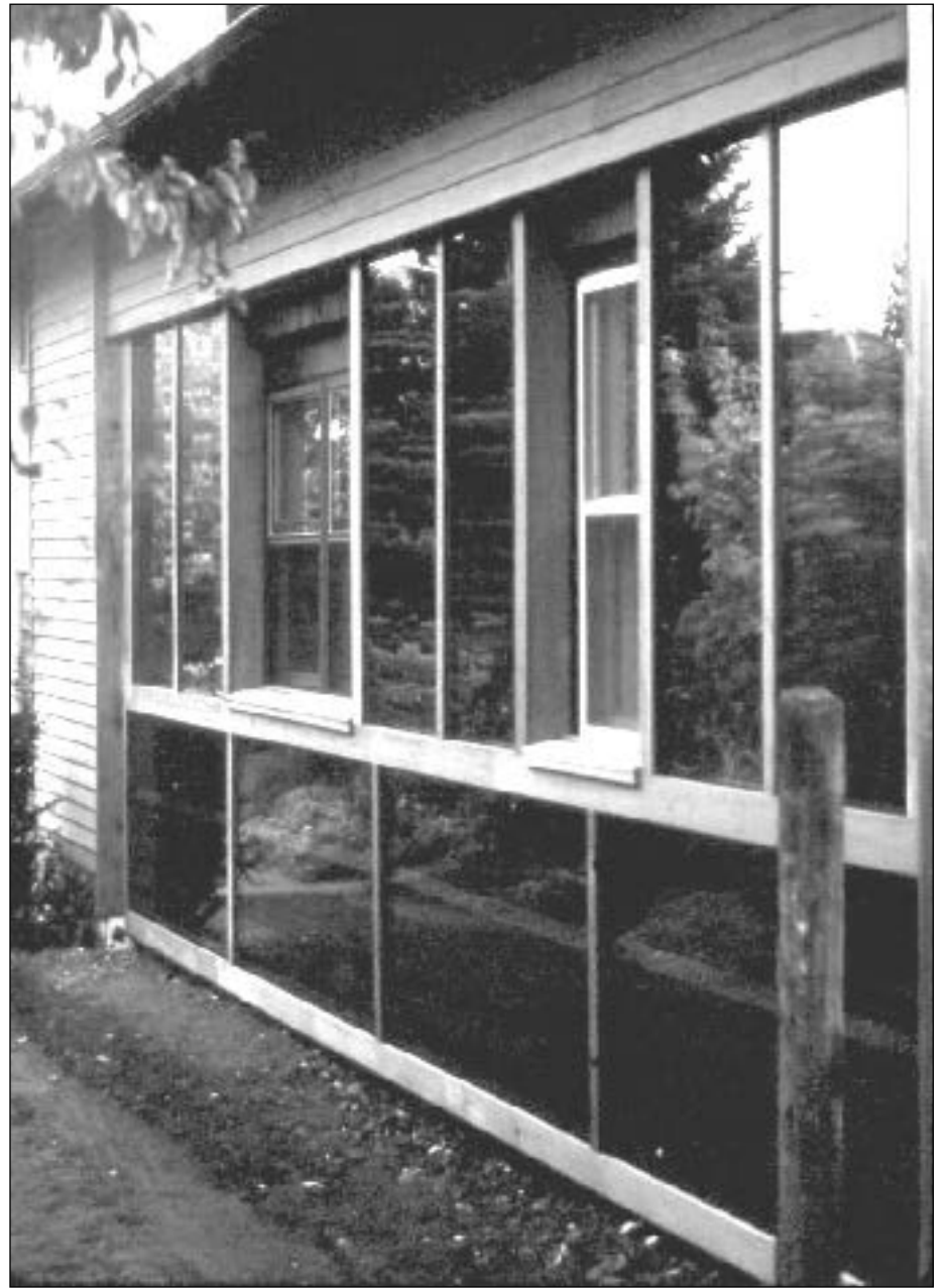
Some century-old brick homes call for installing a glass wall on the south side and wrapping the other three sides with insulation and new siding.
