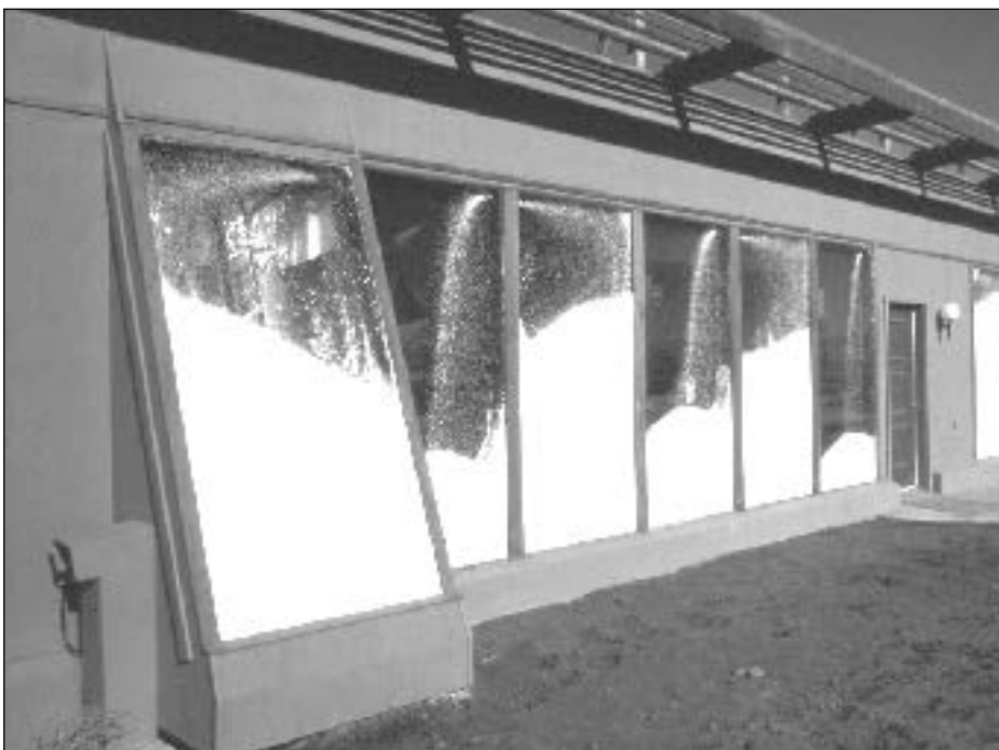
Insulating windows with blinds, shades or drapes is one of the most effective ways of saving energy. Here, styrofoam beads blown between two layers of glass 4" apart can greatly enhance the performance of a passive solar system on winter nights. This SunEarth house is 100% solar heated. The beads are sucked out of the windows in the morning by vacuum cleaner motors and stored in large metal bins in the garage.
